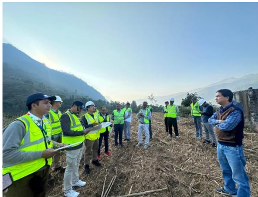
Picture 1: Briefing at Ratmate S/S site
