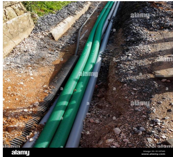
Fig-4, PLHDPE Pipe Laying in Trench
