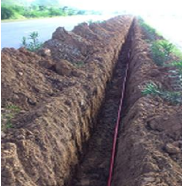
Fig-6, PLHDPE Pipe Laying in Trench
