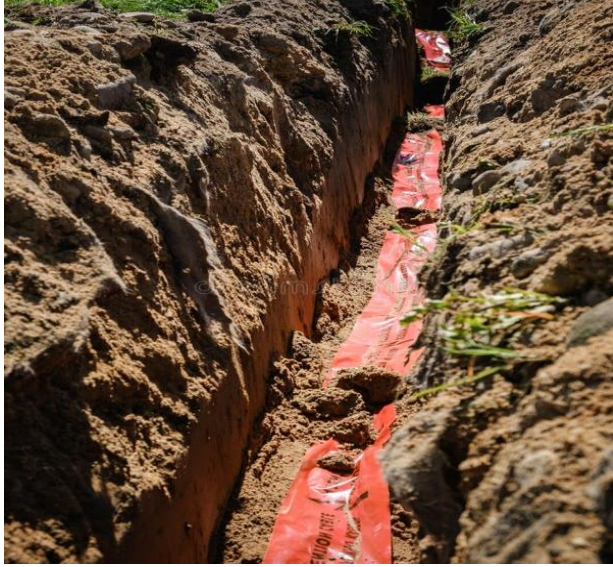
Fig-4, Laying of Warning Tape above PLHDPE Pipe
