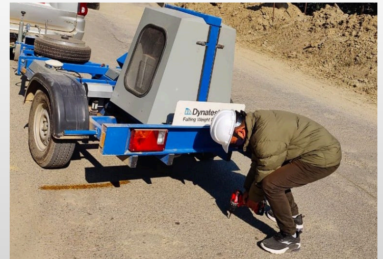
Deflection measurement using FWD
