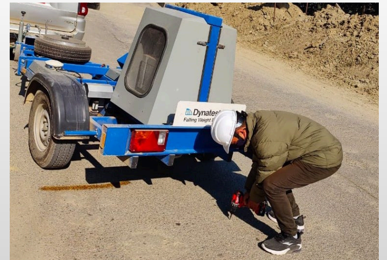
Deflection measurement using FWD
