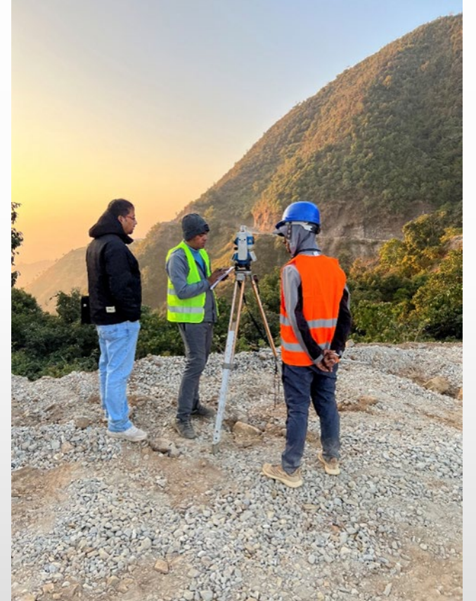
Re-survey work of 30 km
