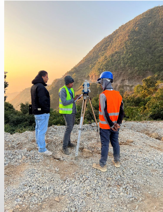
Re-survey work of 30 km
