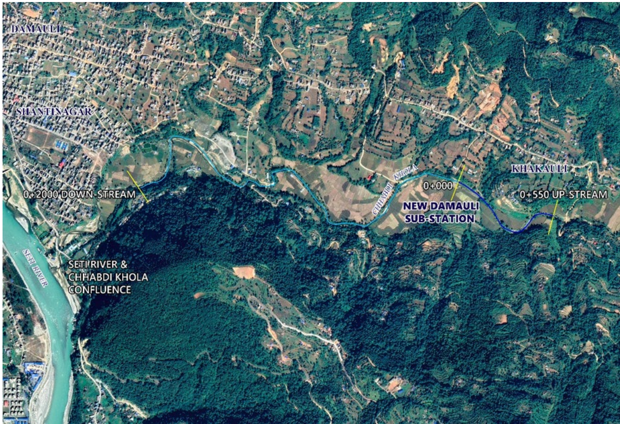
Figure 15-2: Google Image of Substation location
