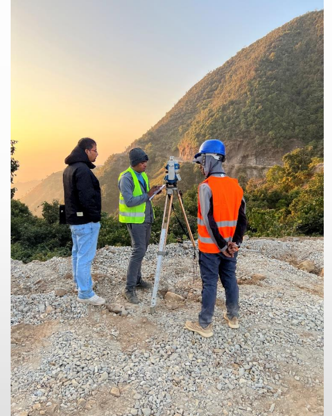
Re-survey work being carried out in Chitwan.
