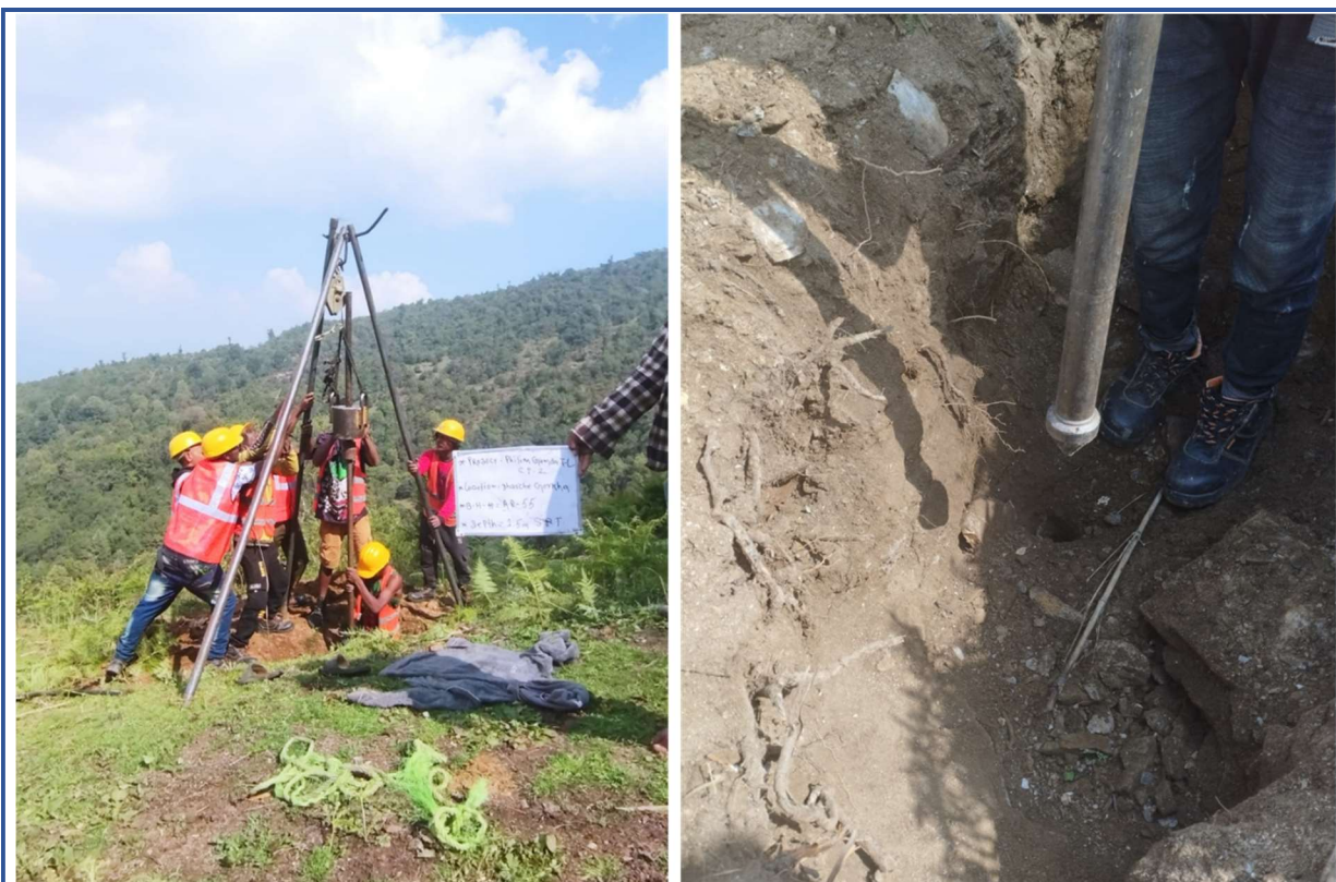
Figure 4-4: Typical DCPT Setup at Site
