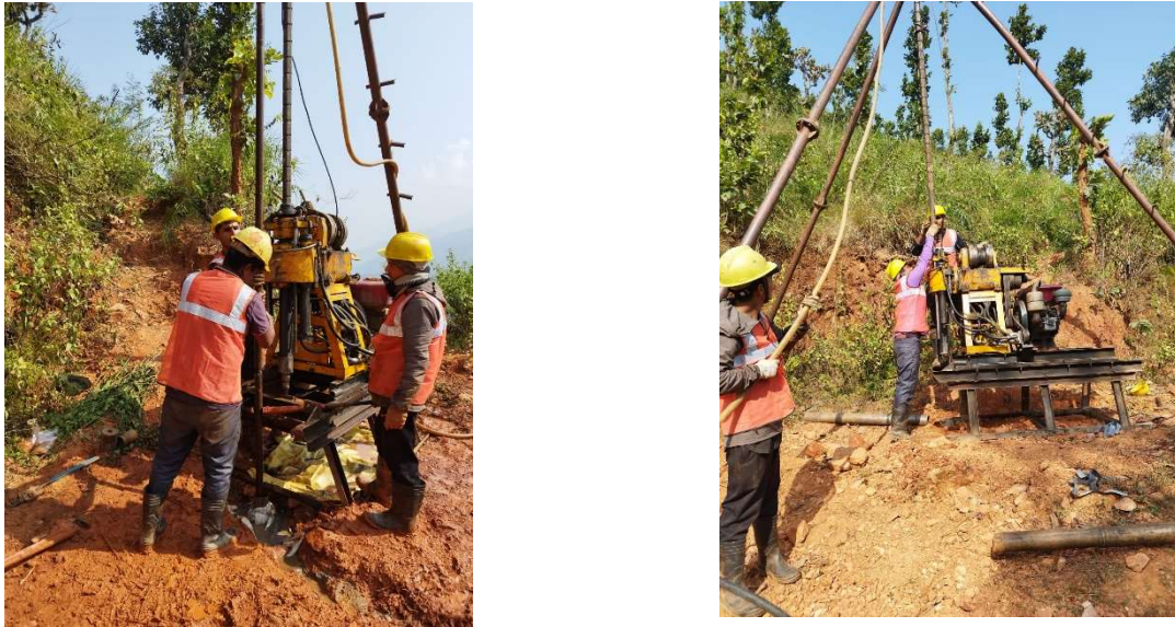
Figure 4-2: Rotary Drilling Method at Nuwakot Section
