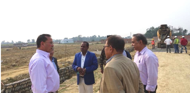
MCA-Nepal with the DCC Chief of Parasi Mr. Shiva Shankhar Ray at New Butwal Substation site.
