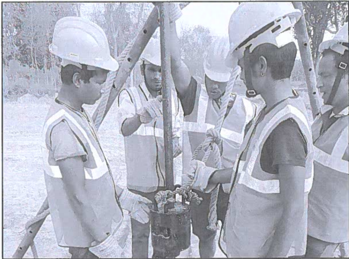
Photograph: Performing SPT test at B3Hole
