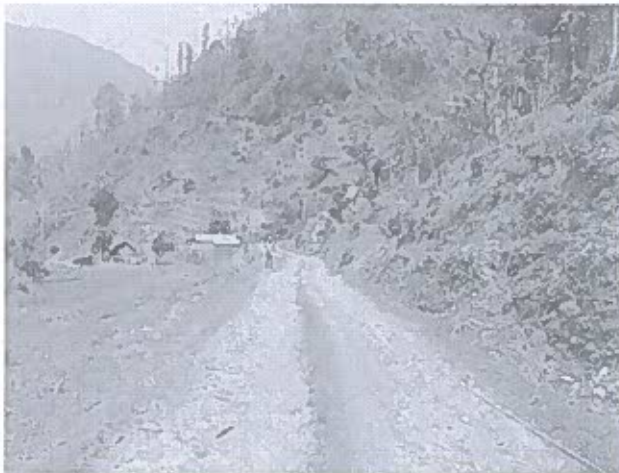
Preparation of profile for soil resistivity test at B56
