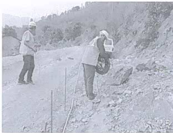
Preparation of profile for soil resistivity test at B36
