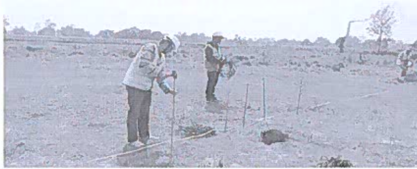
Preparation of profile for soil resistivity test at B5
