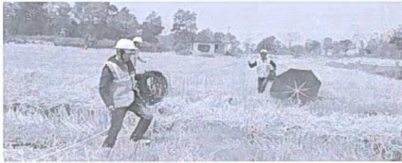
Preparation of profile for soil resistivity test at B3
