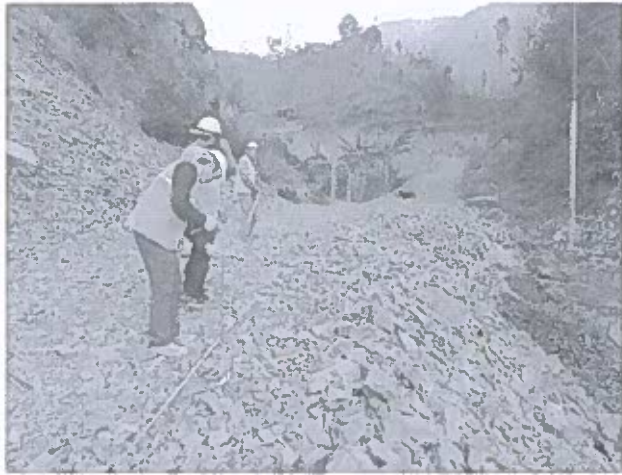
Preparation of profile for soil resistivity test at B30
