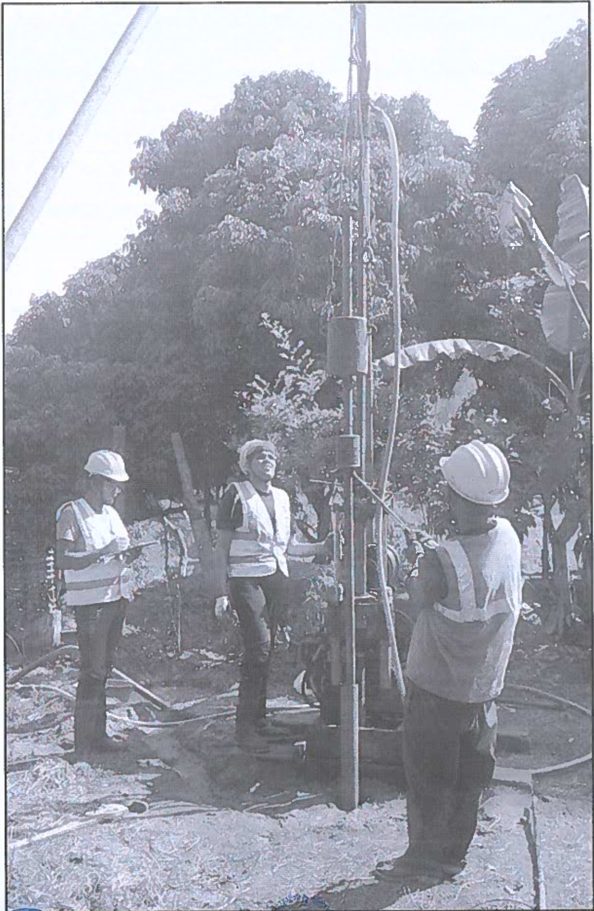
Photograph: Performing SPT test at B34
