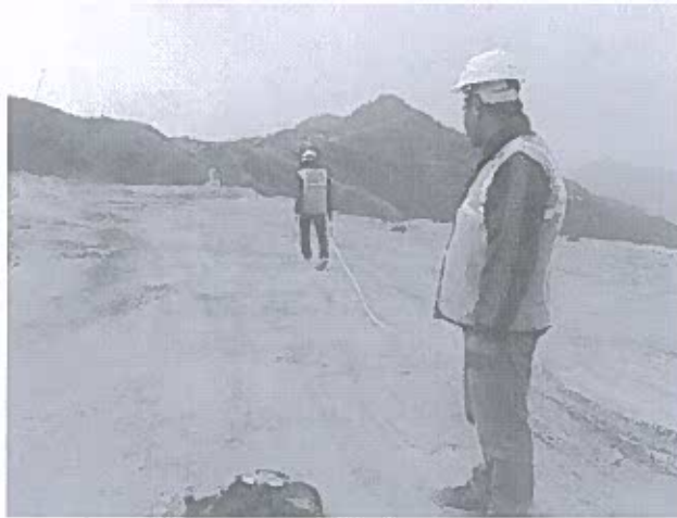
Preparation of profile for soil resistivity test at B54
