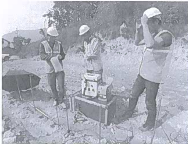
Preparation of profile for soil resistivity test at B58
