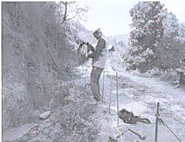
Preparation of profile for soil resistivity test at B47
