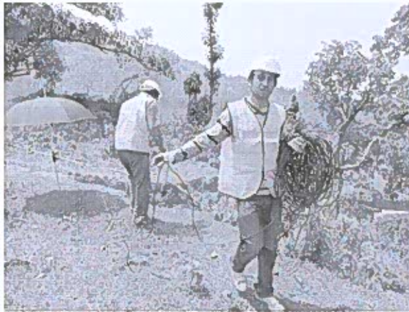
Preparation of profile for soil resistivity test at B15
