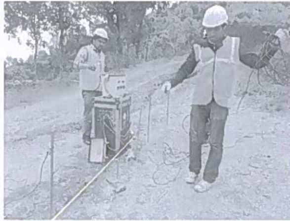
Preparation of profile for soil resistivity test at B20
