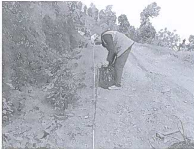
Preparation of profile for soil resistivity test at B40
