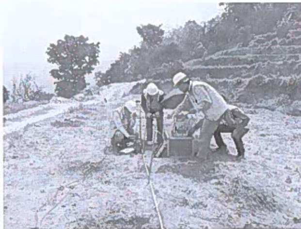
Preparation of profile for soil resistivity test at B41
