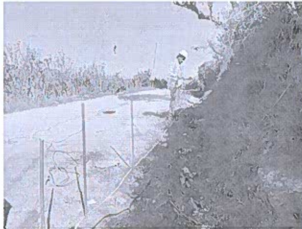
Preparation of profile for soil resistivity test at B25
