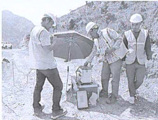
Preparation of profile for soil resistivity test at B31
