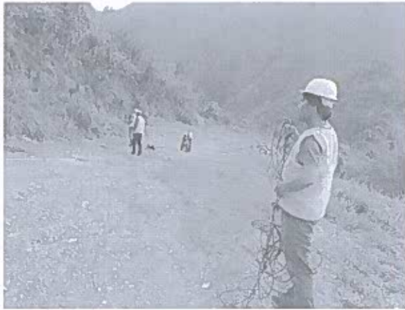
Preparation of profile for soil resistivity test at B22
