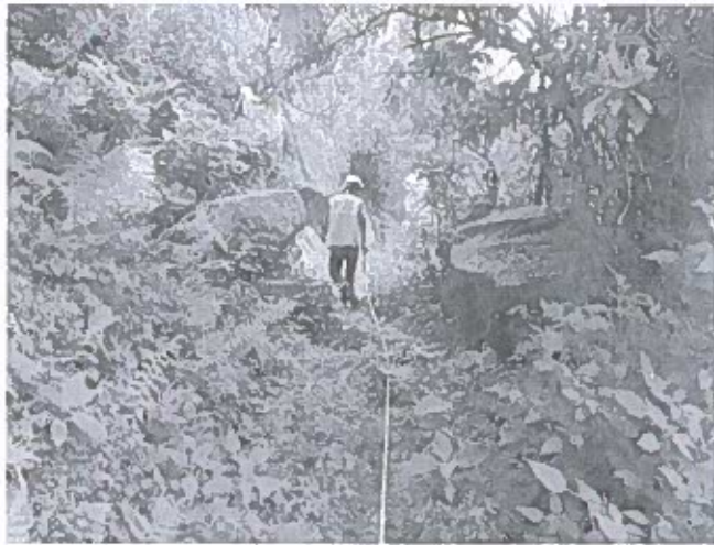
Preparation of profile for soil resistivity test at B46
