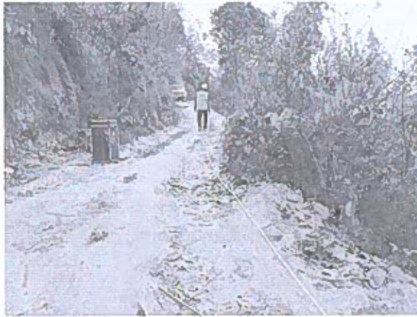
Preparation of profile for soil resistivity test at B43
