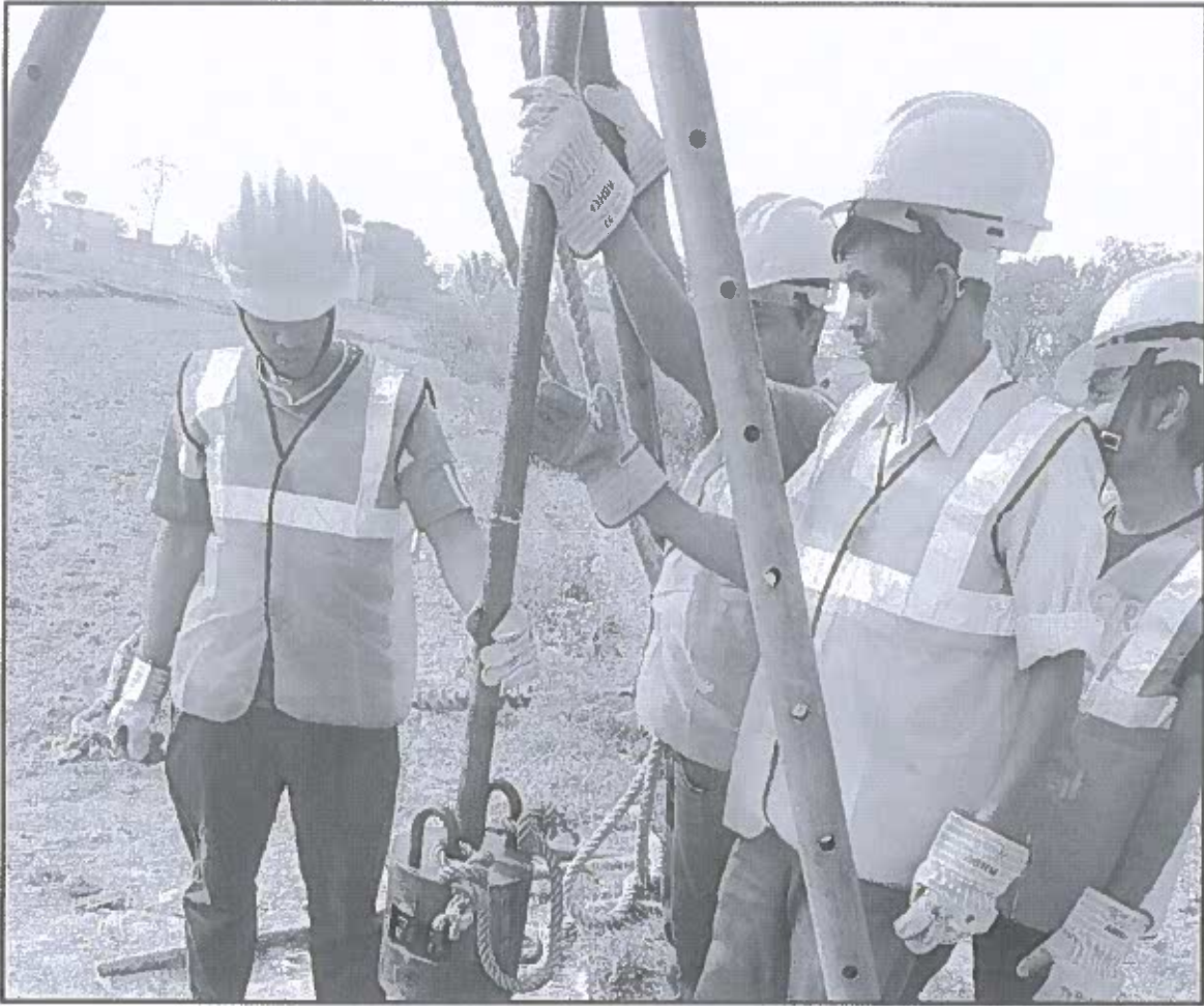
Photograph: Preparatory setup for the SPT test at B6 Hole
