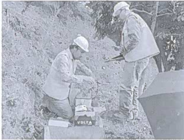
Preparation of profile for soil resistivity test at B18
