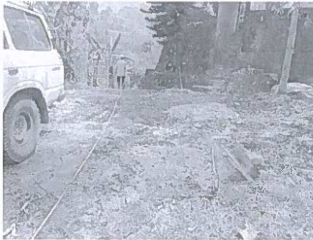
Preparation of profile for soil resistivity test at B34
