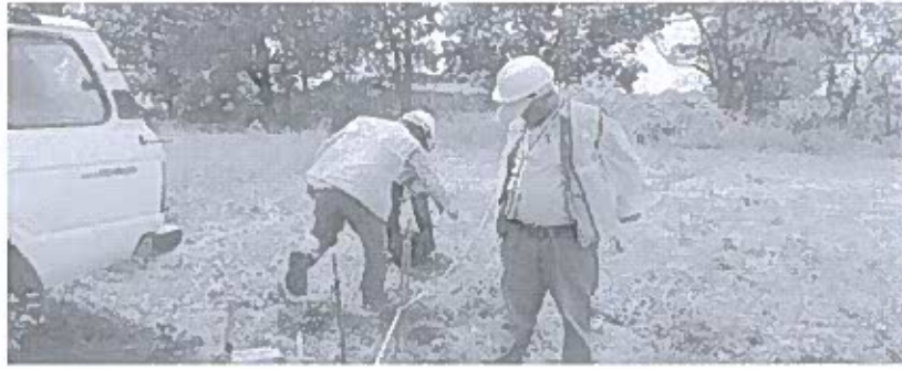
Preparation of profile for soil resistivity test at B4
