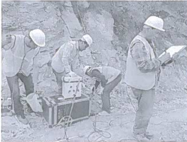
Preparation of profile for soil resistivity test at B32
