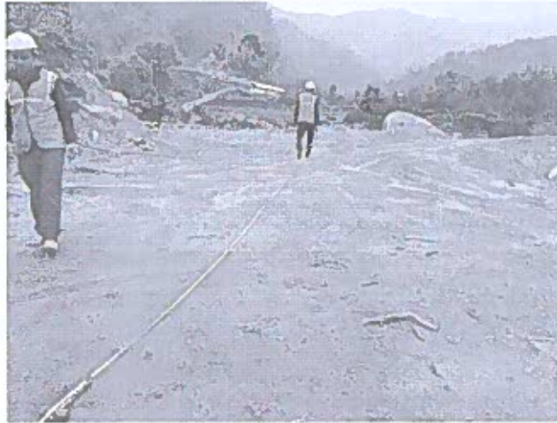
Preparation of profile for soil resistivity test at B55
