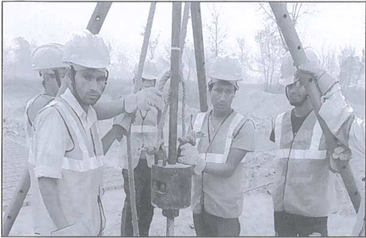
Photograph: Performing SPT test at B4Hole
