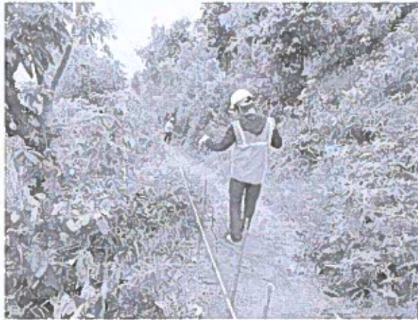
Preparation of profile for soil resistivity test at B19
