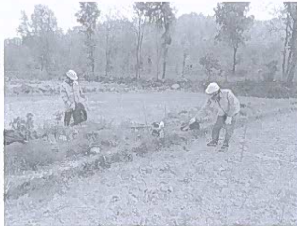
Preparation of profile for soil resistivity test at B10
