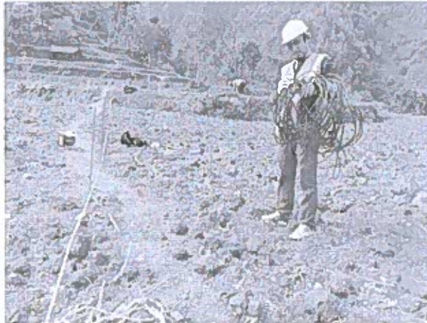
Preparation of profile for soil resistivity test at B21
