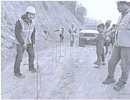
Preparation of profile for soil resistivity test at B13
