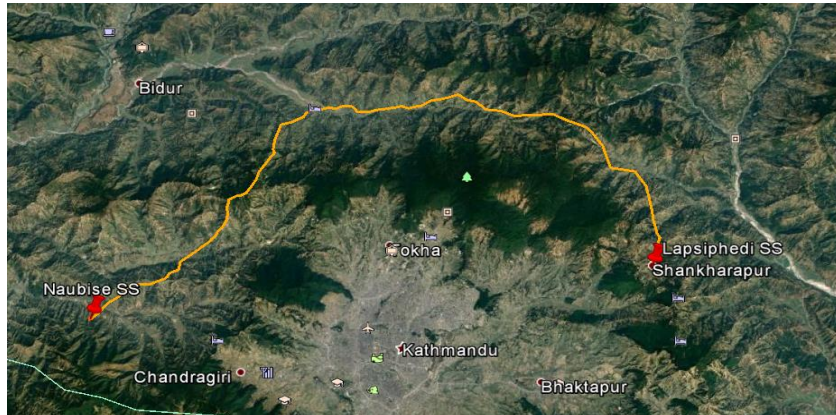
Figure 2.9 NR1- Naubise to Lapsipedi 400 kV Transmission Line
