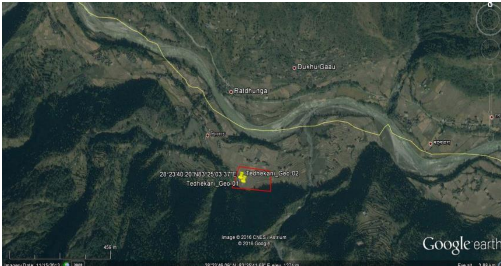
Figure 2.5.4.17: Tadhekani Substation (Zoom Out)
