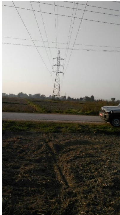
Figure 3.41 132 kV Line on Future Site for New Butwal Station
