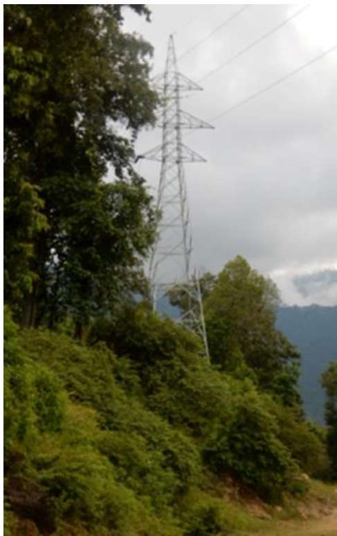
Figure 45. Transmission Towers and Trees along the Existing NR4 Project Route
